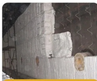
Furnace insulation
