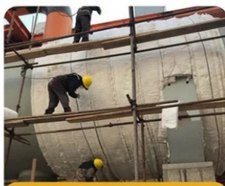
Tank insulation
