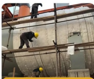
Tank insulation
