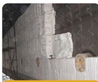
Furnace insulation
