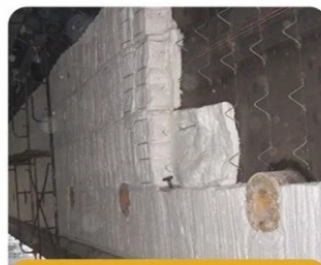
Furnace insulation
