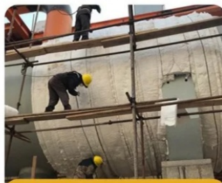
Tank insulation
